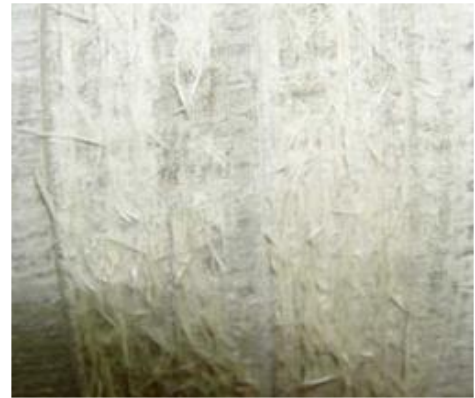
Figure 1. Example of a surface defect - fraying resulting from the cutting of reinforcing fibers.
