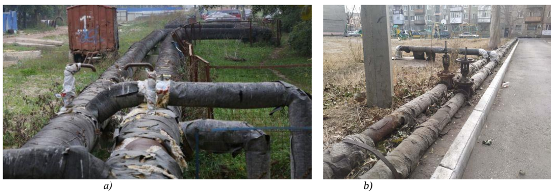
Figure 1. Heat loss in pipes.
